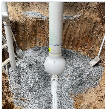
Kerkin Adventure Park Water cut-in for dual water meters
