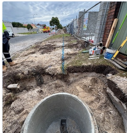
2 Biota Ct Sewer main extension for IO
