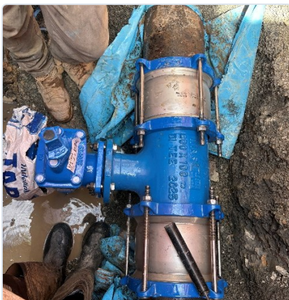
19 Nangana St Sewer extension on lot
