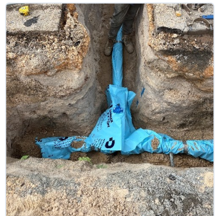
111 Hedges Ave Water cut-in for above ground meter
