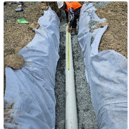
Stadium Drive Sewer main extension w/ manholes
