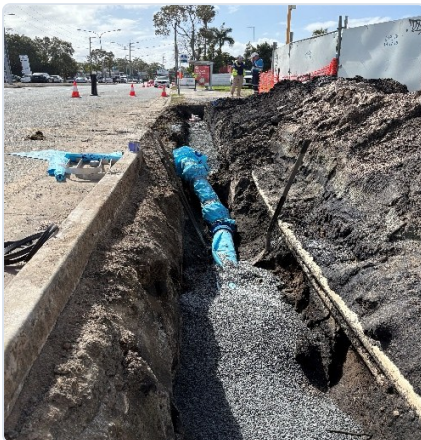
278 Ferry Road Water main upgrade
